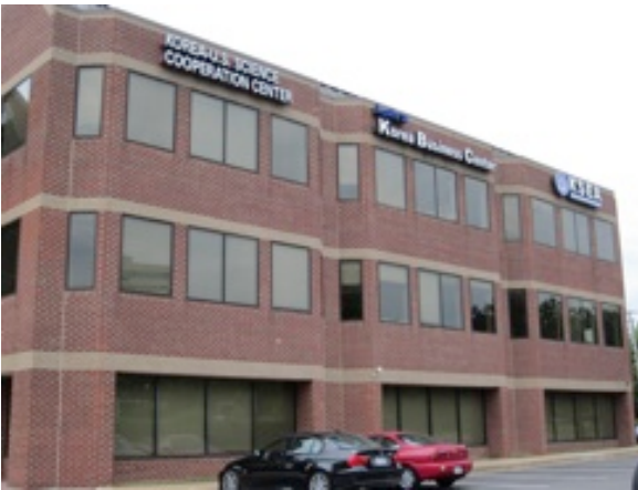
Fig. 1: KUSCO/KSEA building, Vienna, VA
